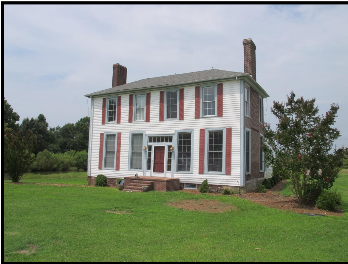
Figure 20: Sumner-Winslow House (# 2), Looking Southwest.
