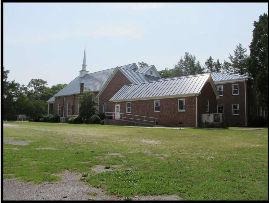
Figure 7: Ballard's Bridge Baptist Church (# 1), Looking Southeast.
