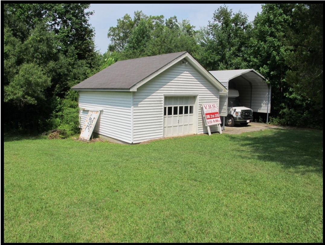
Figure 16: Ballard's Bridge Baptist Church (# 1), Garage and Carport, Looking West.
