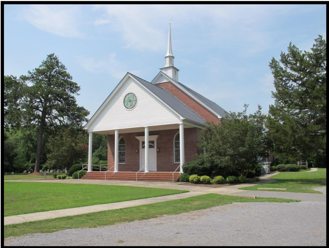
Figure 6: Ballard's Bridge Baptist Church (# 1), Looking Southwest.
