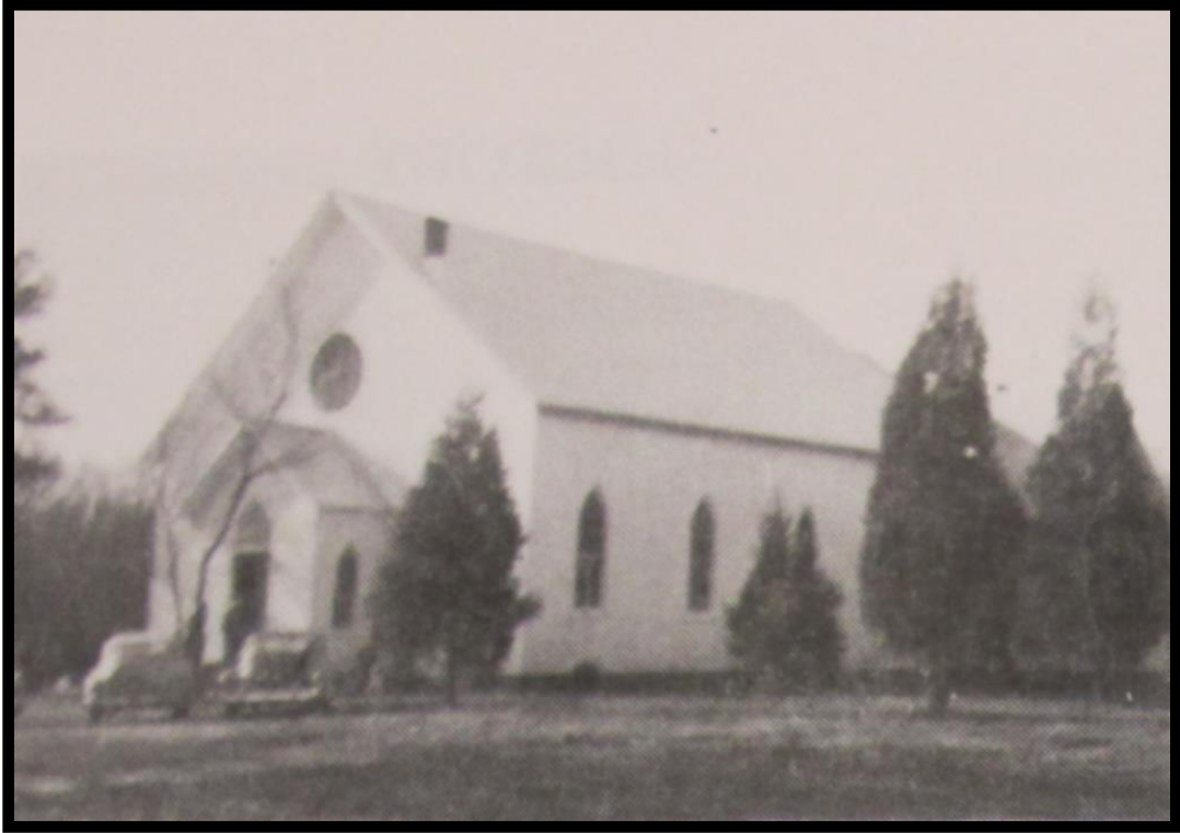
Figure 5: Historic Photograph of Ballard's Bridge Baptist Church (# 1), Looking Southwest (prior to 1950).
