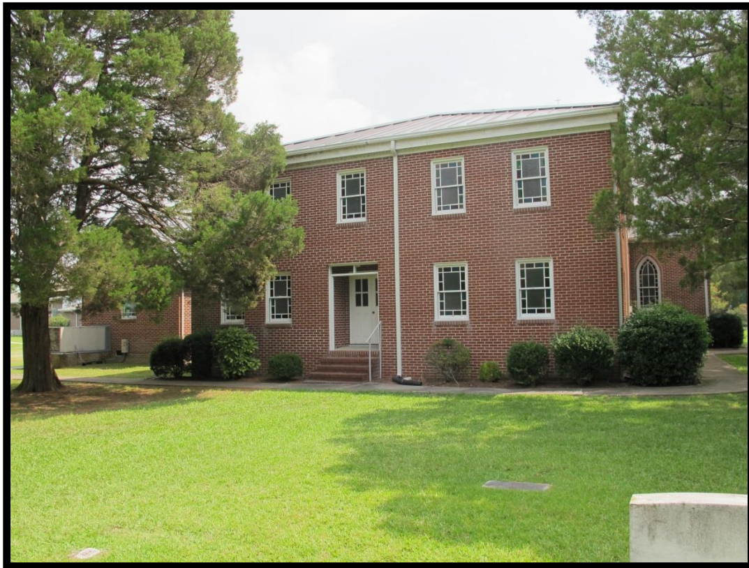
Figure 8: Ballard's Bridge Baptist Church (# 1), Looking Northeast.
