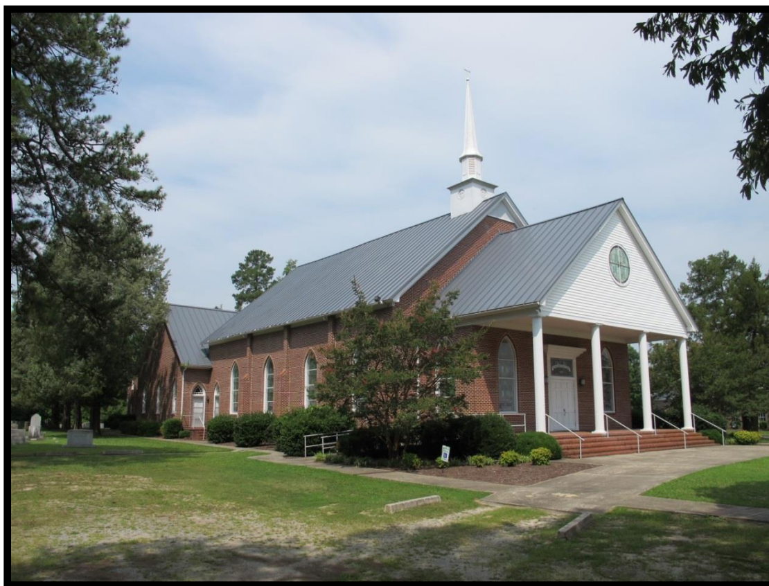
Figure 3: Ballard’s Bridge Baptist Church (# 1), Looking Northwest.
