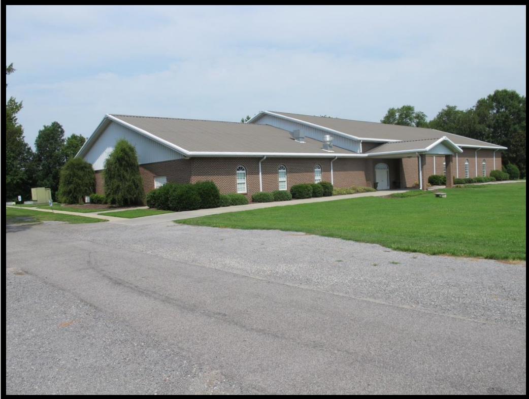
Figure 17: Ballard's Bridge Baptist Church (# 1), Fellowship Hall, Looking Northwest.
