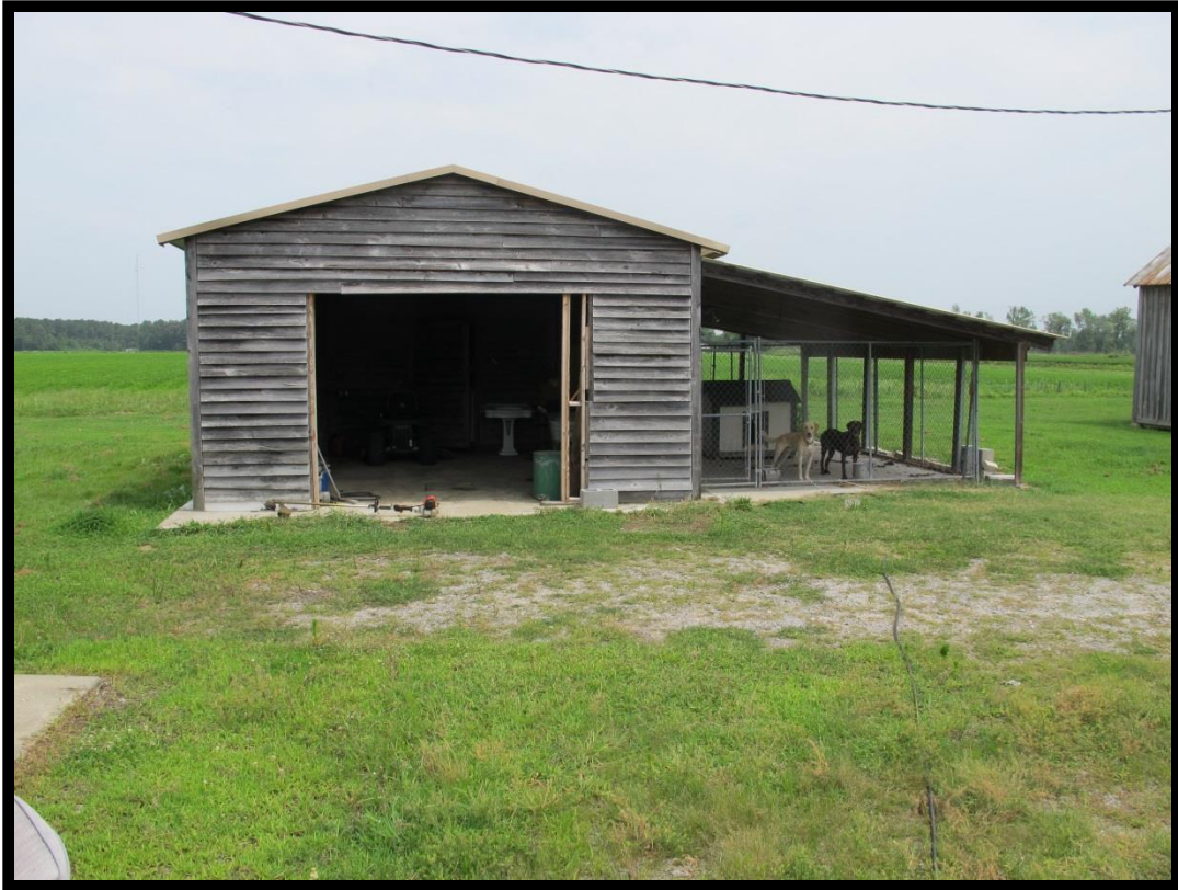
Figure 29: Sumner-Winslow House (# 2), Garage/Kennel Looking North.
